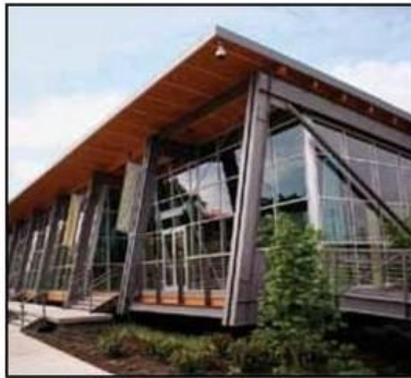
Figure 3: The Discovery Center, South Lake Union, Seattle, WA designed by The Miller|Hull Partnership with Magnusson Klemencic Associates as structural engineer. Courtesy of Magnusson Klemencic Associates.
