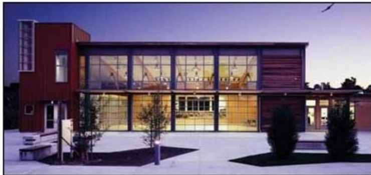
Figure 1: The Chartwell School, Seaside, CA, designed by EHDD Architecture with Tipping + Mar Associates as structural engineer. Courtesy of Michael David Rose / MDRP.NET.
